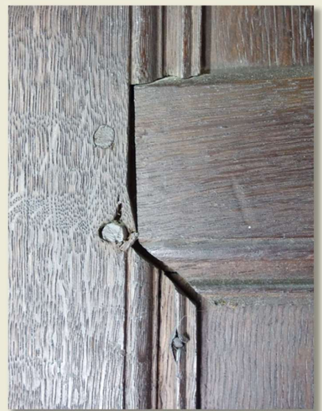
Distortions in Paneling W side of N I
