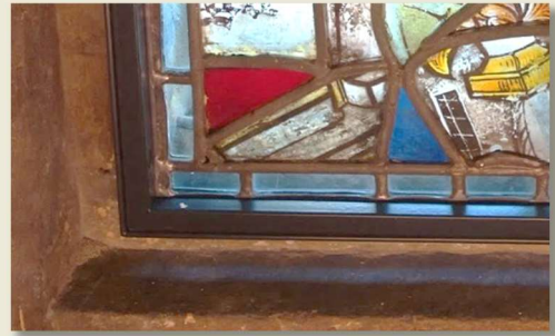
Conserved glass in new metal frames
